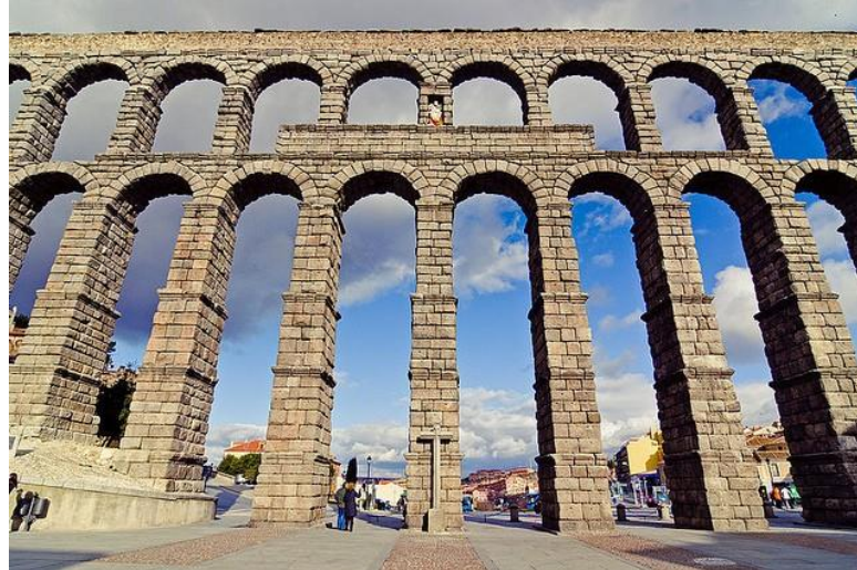
Fig.2. Aqueduct of Segovia, Spain.
