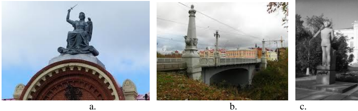
Fig.1. a) Nemesis, the building of the District Court, architect K.K. Lygin, 1904 b) stone bridge on Rosa Luxemburg Street, architect K.K. Lygin, 1916 c) monument to V.V. Kuibyshev, University grove of TSU, 1990s
